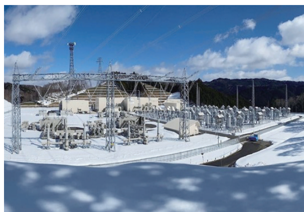
Chubu Electric Power Grid Hida Shinano Frequency Conversion Facility: Hitachi delivered a high-voltage direct current (HVDC) system to this facility. Hitachi Energy products are used in the AC filters.
